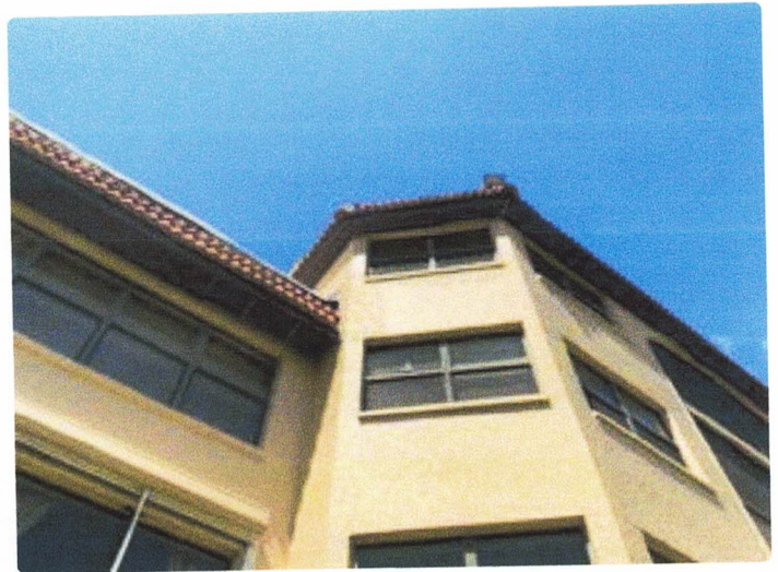
Missing soffit
