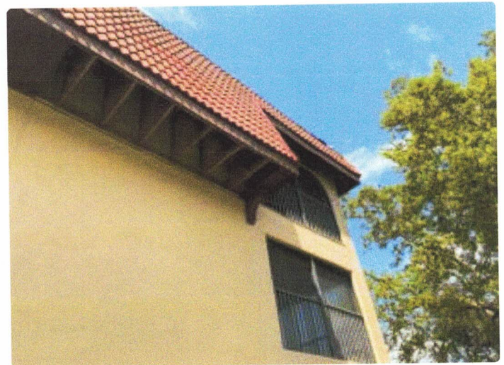
Missing soffit
