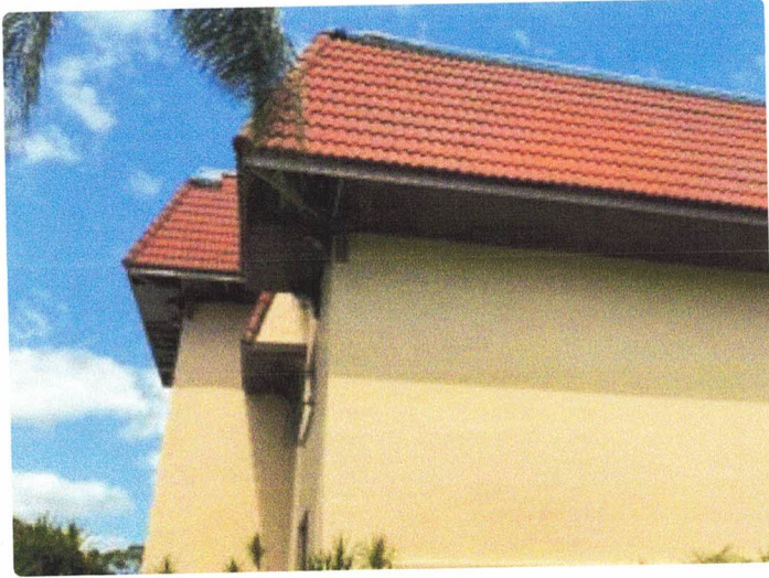
Missing soffit
