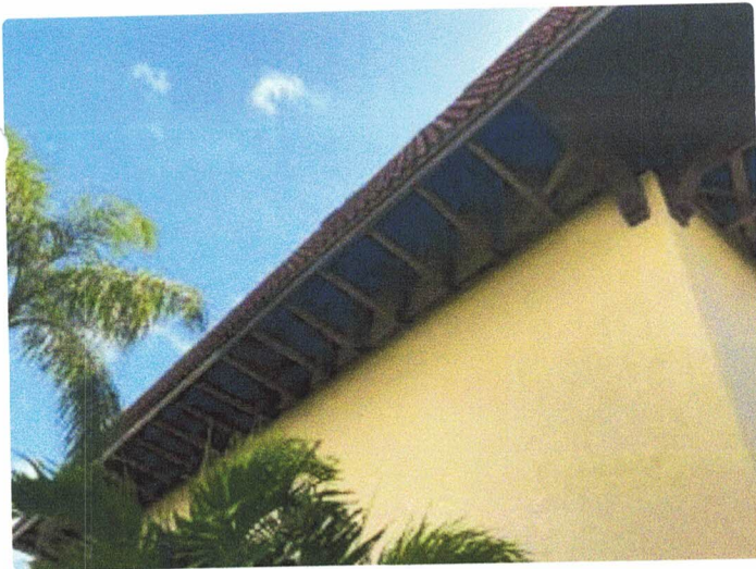
Missing soffit
