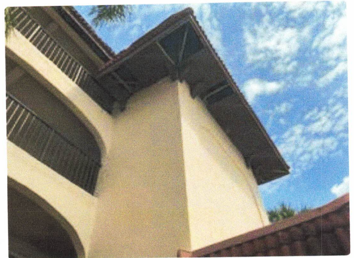
Missing soffit
