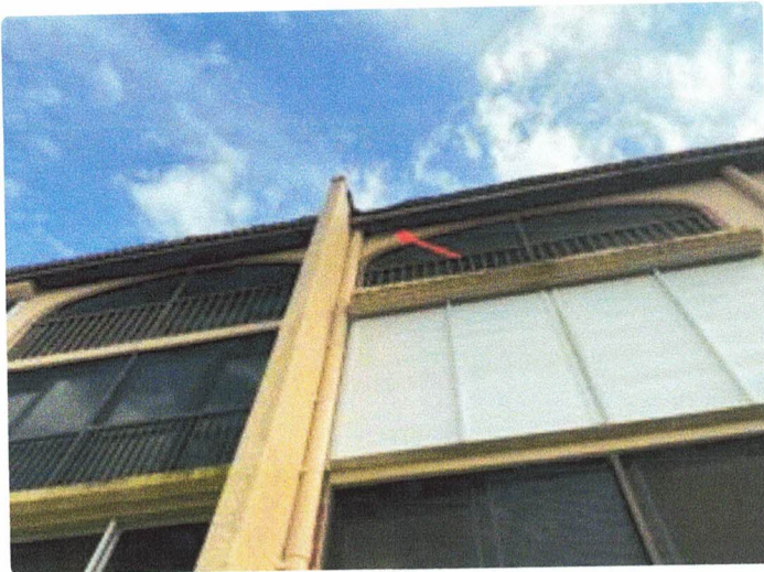
Missing soffit
