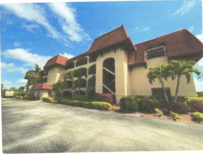
Typical exterior wall
