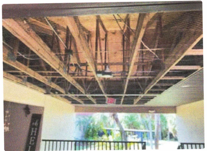
Missing soffit
