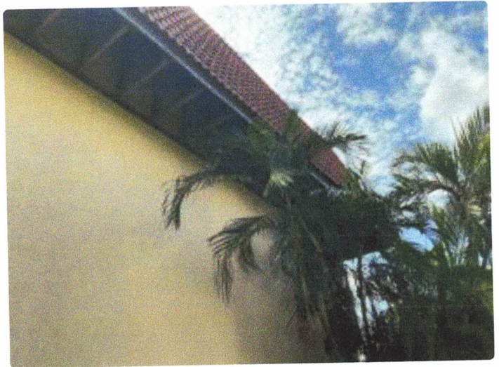
Missing soffit
