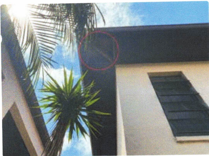
Missing soffit
