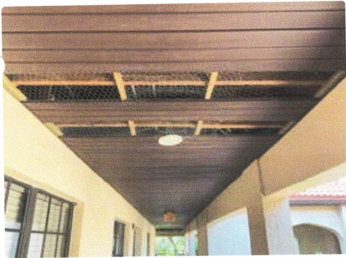
Missing soffit
