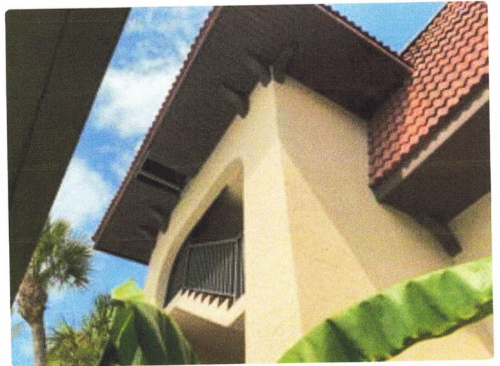
Missing soffit
