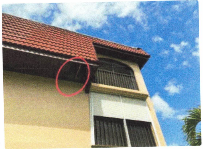
Missing soffit
