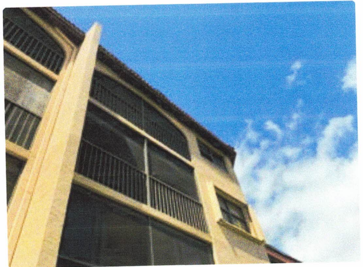
Missing soffit
