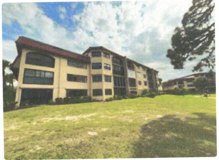
Typical exterior wall
