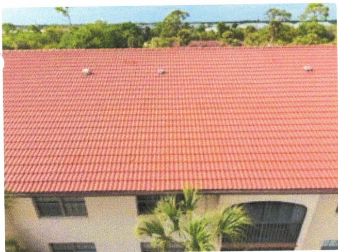
Broken barrel tiles
