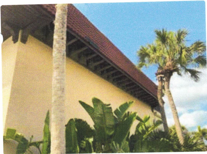
Missing soffit
