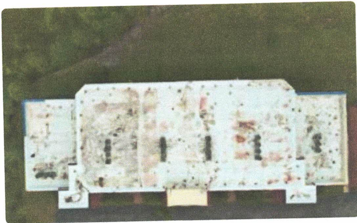
Typical remediation overview
