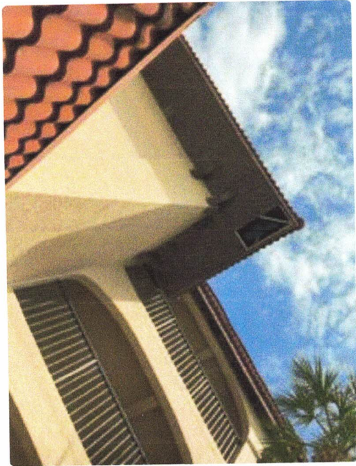
Missing soffit
