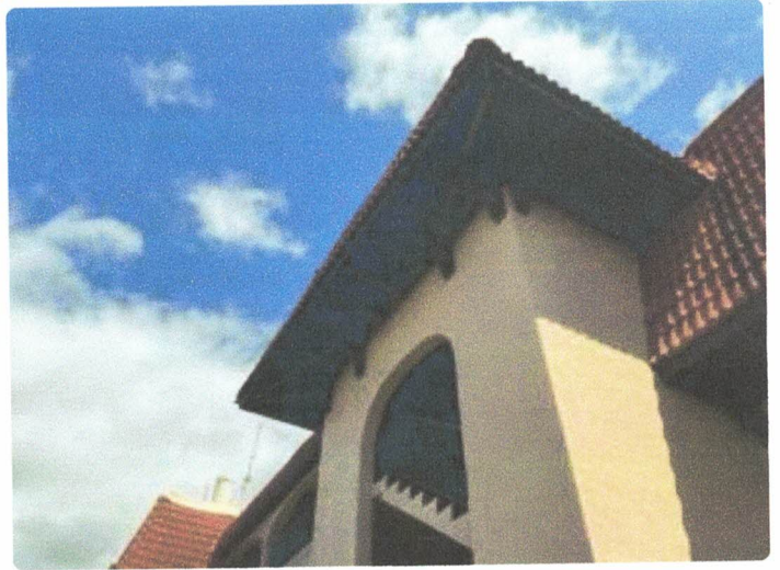
Missing soffit
