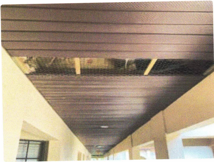
Missing soffit
