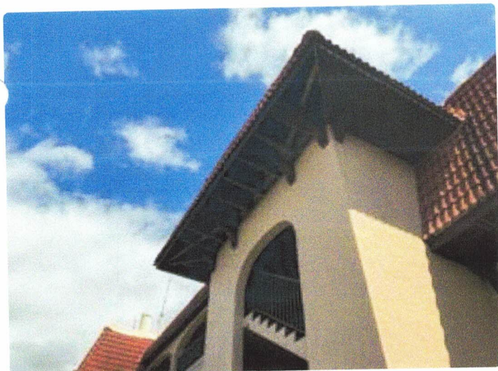
Missing soffit
