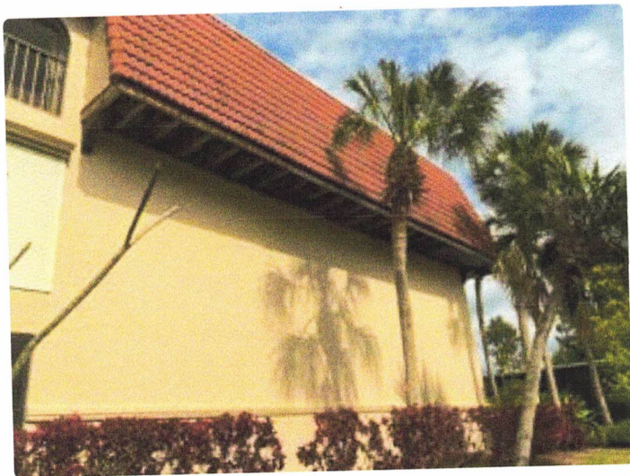
Missing soffit
