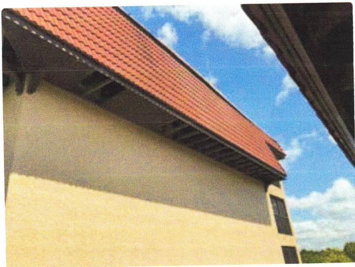
Missing soffit
