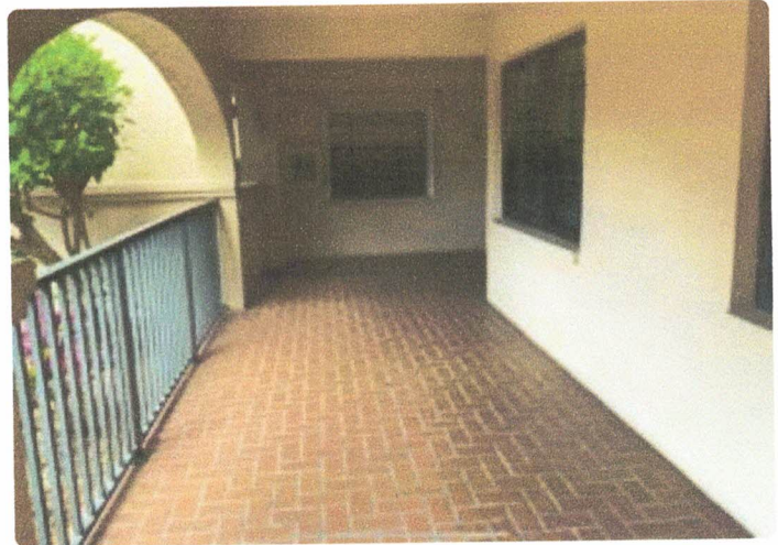
First level floor
