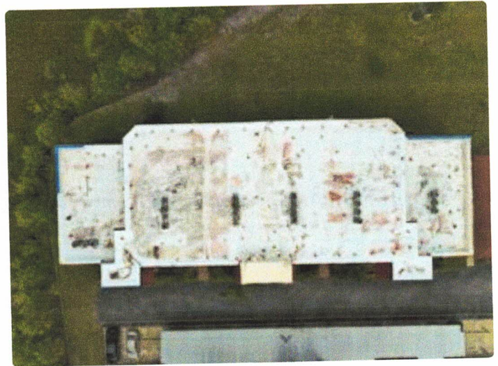
Temporary remediation on roof
