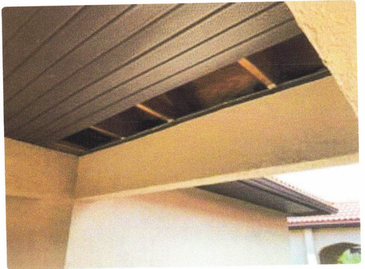
Missing soffit
