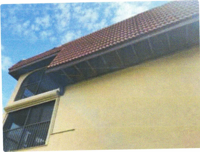
Missing soffit
