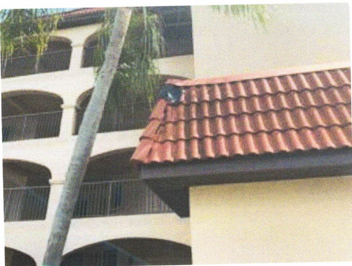
Remedial fix on broken barrel tile
