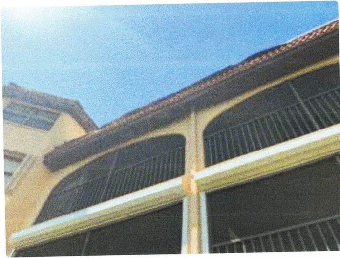
Missing soffit
