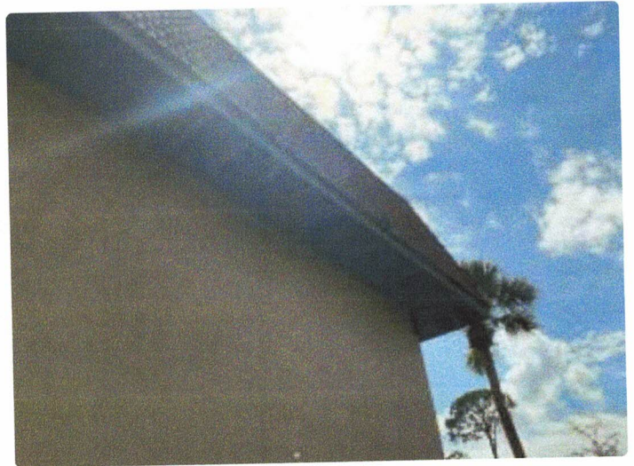
Missing soffit
