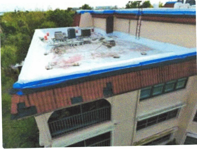
Barrel tile remediation
