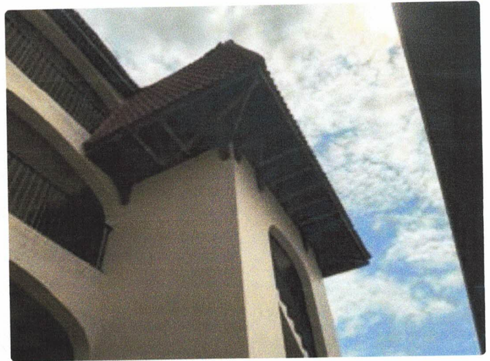
Missing soffit
