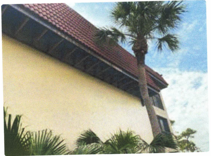
Missing soffit
