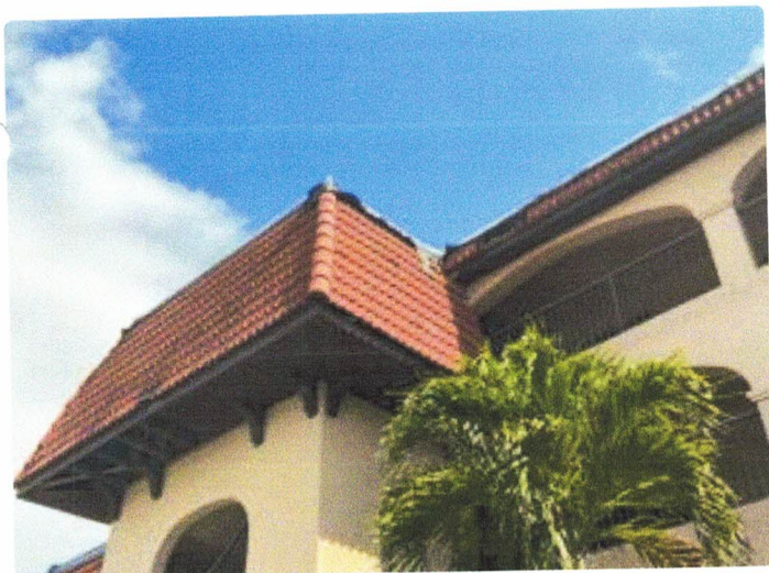
Remedial fix on broken barrel tiles
