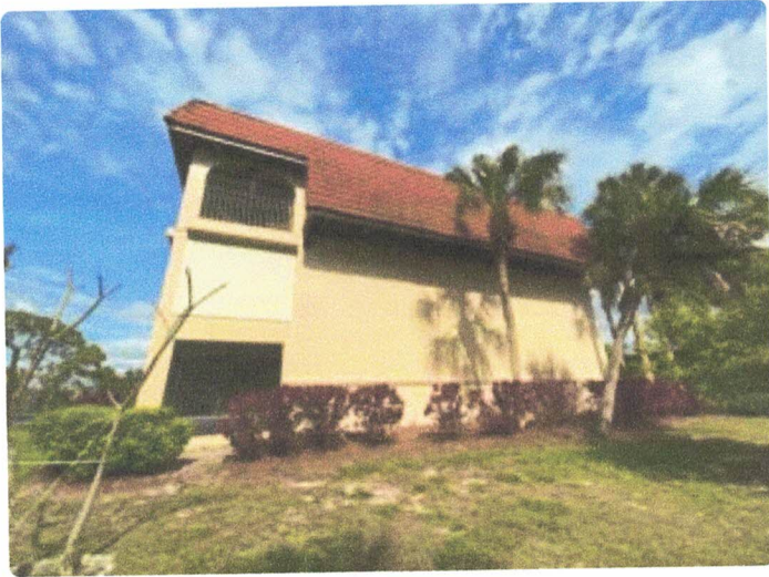
Typical exterior wall
