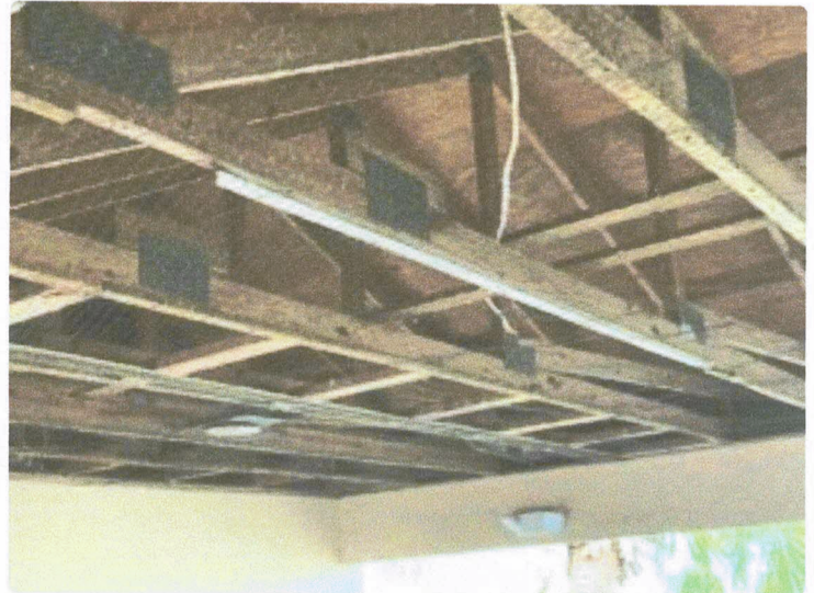
Trusses from second floor.
