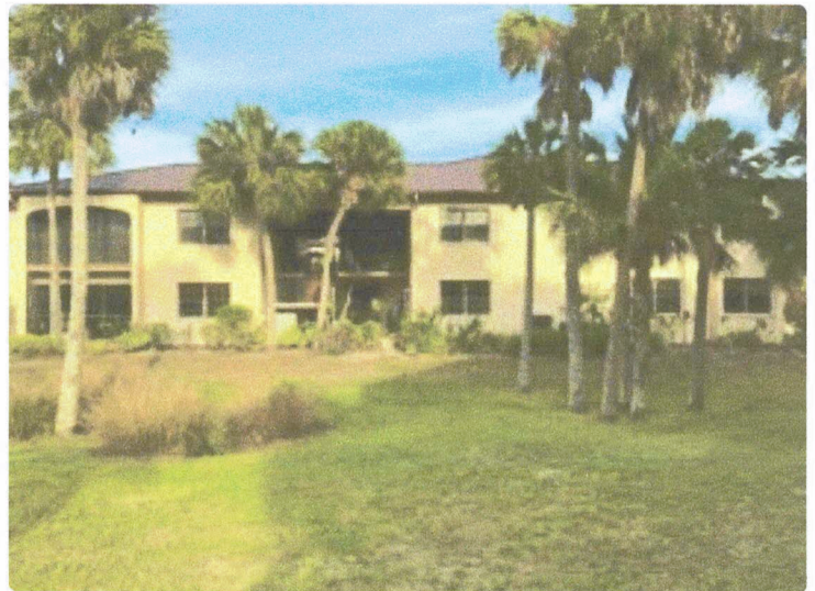
Right Elevation photo.
