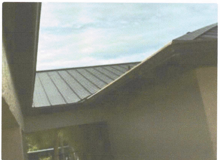
Second floor overview photo of metal roof.
