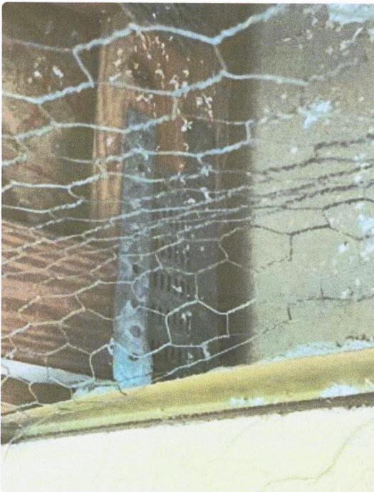
8 nails used to set strap.
