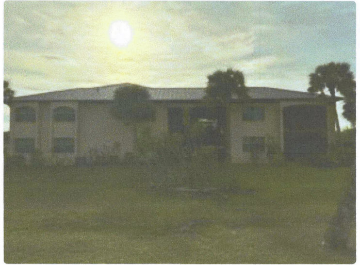
Left Elevation photo.
