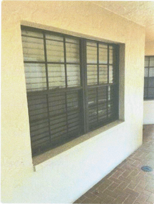
Non impacted window. Level X glazed opening.
