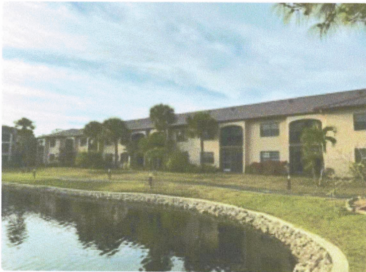
Rear elevation photo of roof.
