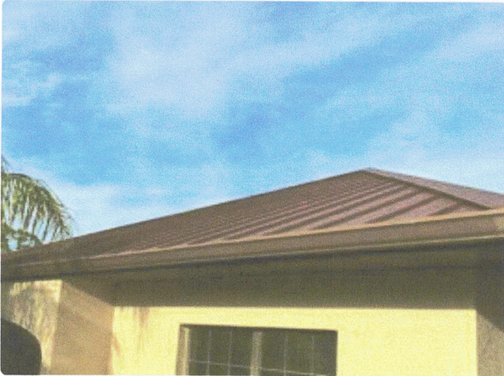
Second floor photo of metal roof.
