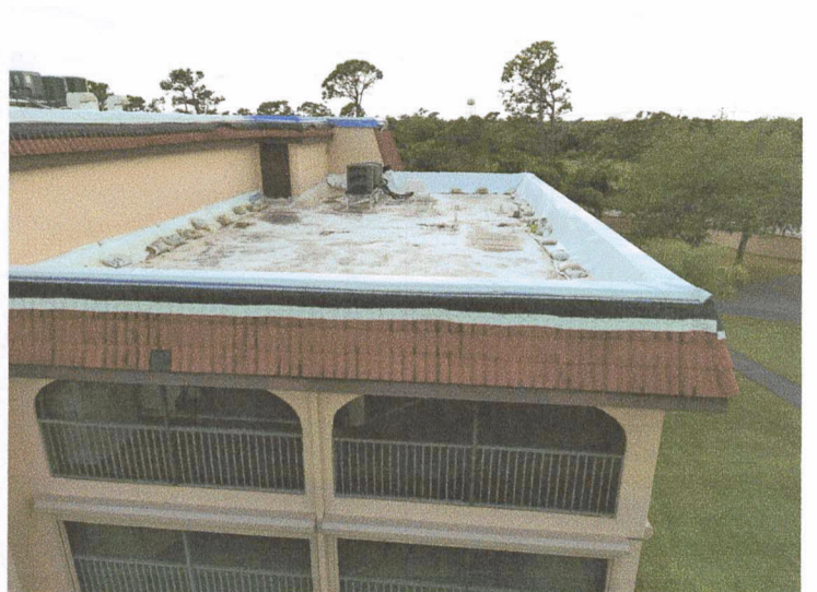
Tarped parapet post lan
