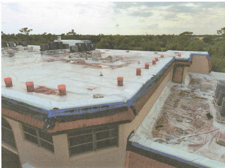
Tarped roof post lan
