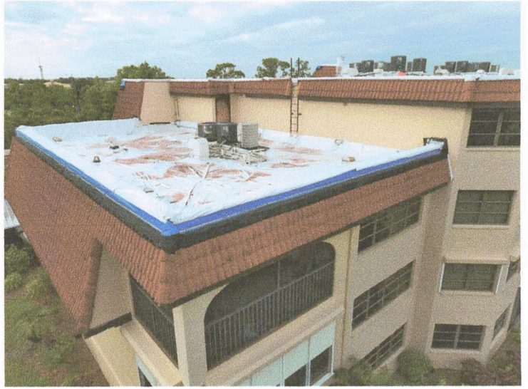
Tarped roof post lan
