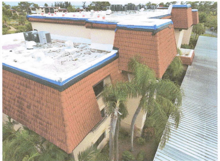
Tarped roof post lan
