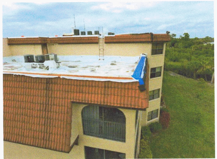
Tarped roof after Ian
