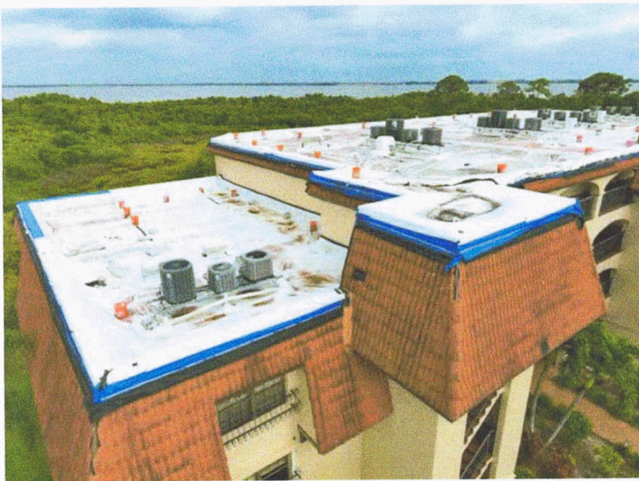
Tarped roof after Ian
